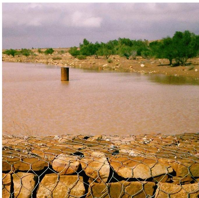
A recharge well needs to be always combined with a gabion check dam which prevents floodwater movement downstream and creates a temporary pond (Temmerman S.)
