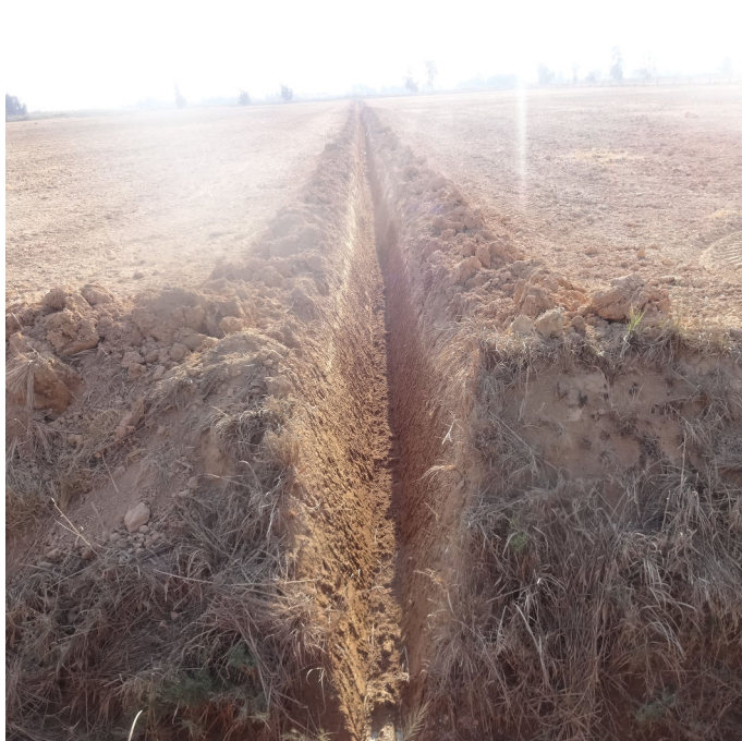
Drainage ditch constructed in a field with a problem of drainage and high calcium carbonate content. (Daniel Danano Dale)
