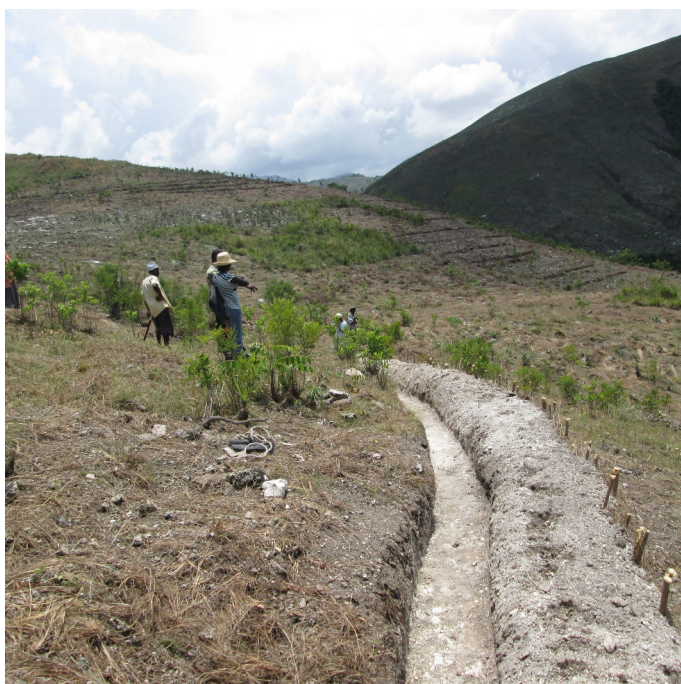
Erosion control structures
