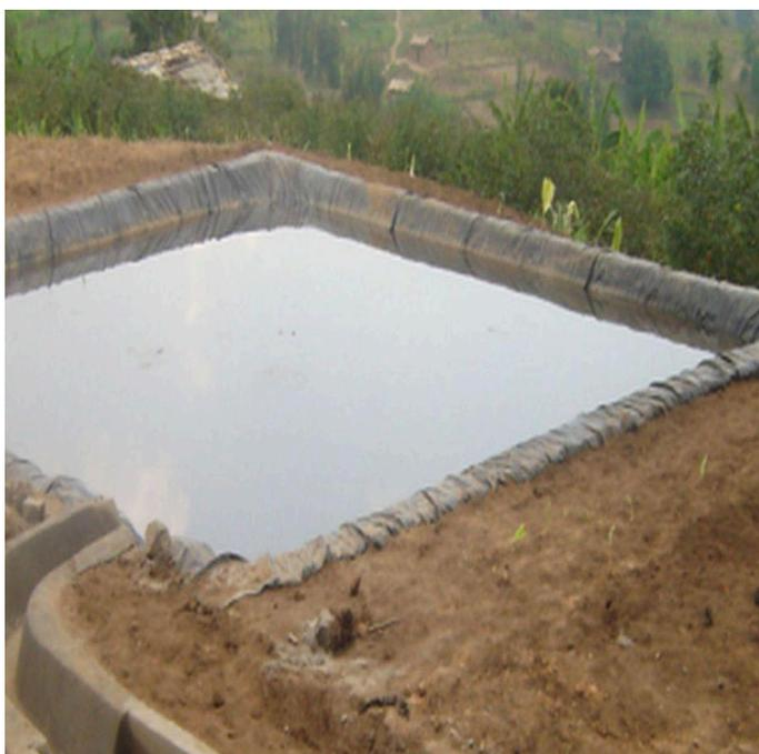
A lining geomembrane plastic is used to stop infiltration of the stored water into the soil (Kagabo Desire and Ngenzi Guy (Kabarondo))
