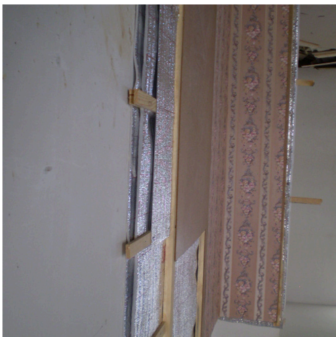
Thermo insulation of room by using foil (Zevvarshoev Askarsho)
