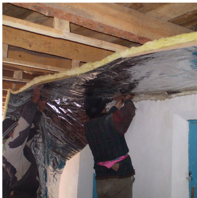
Training for local masters on thermo-insulation of ceiling (Khujiayor Khumorikov)
