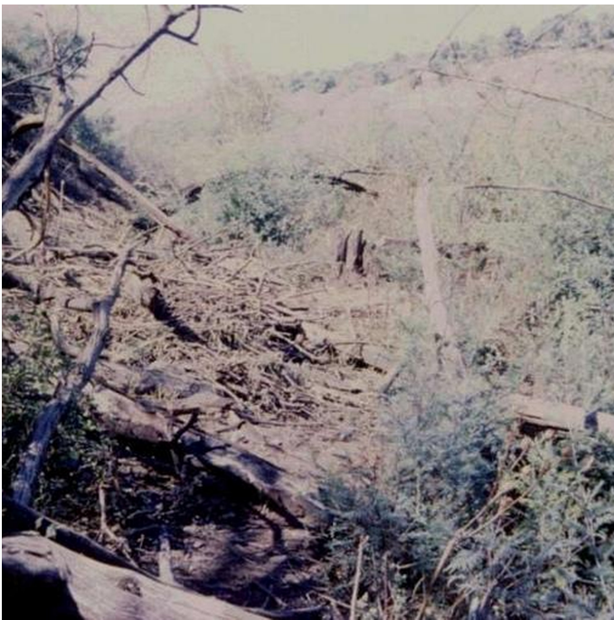
Stacking of heap of pile wood to prevent donga formation into the stream that is densely overgrown by re-growth presently on the right (Schalk Meyer)
