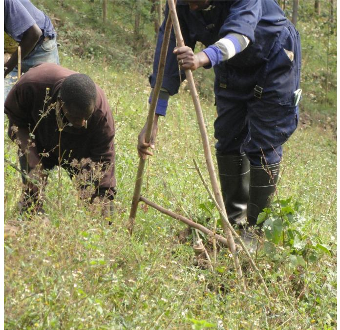
Use of the 'A-frame' to set out the soil and water conservation channels (Kenneth Twinamasiko)
