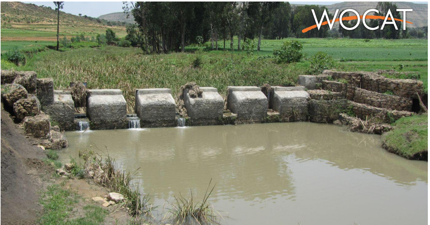
Checkdam with sluice gates removed during rainy season (Eyasu Yazew (Mekelle University, P.O.Box 231, Mekelle, Ethiopia))
