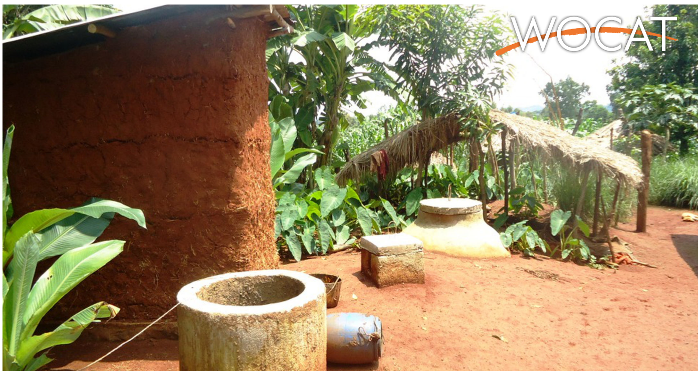
Biogas structure with feedstock from livestock manure and human toilet. (Gerba Leta)
