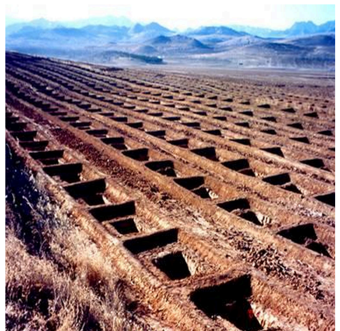
Close view of contour trench (Zhou Xiaole)
