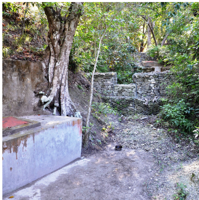
Physical protection of a water intake point
