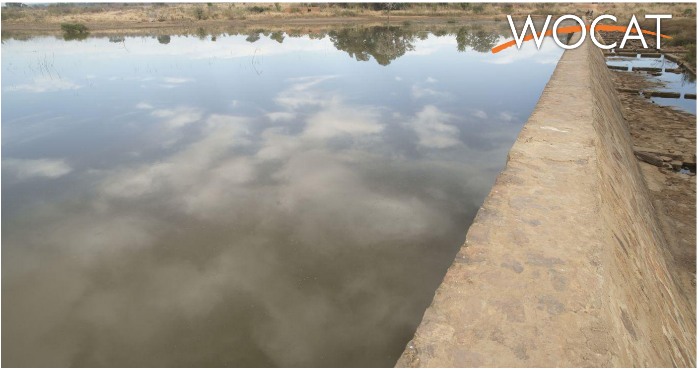
Sounikéyini micro-dam in cyclopean concrete (IPRO-DB)
