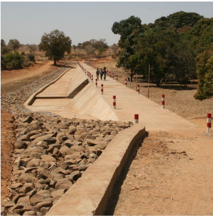
Tiembougou dam bridge in cyclopean concrete (IPRO-DB)
