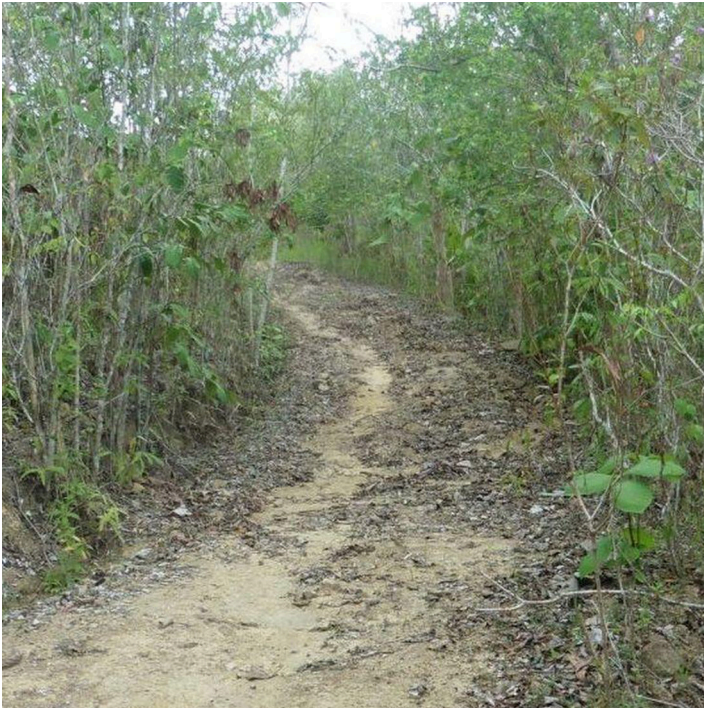
Firebreak with a width of six meters that serves as road network (Engr. Djolly Ma. P. Dinamling (Bureau of Soils and Water Management))
