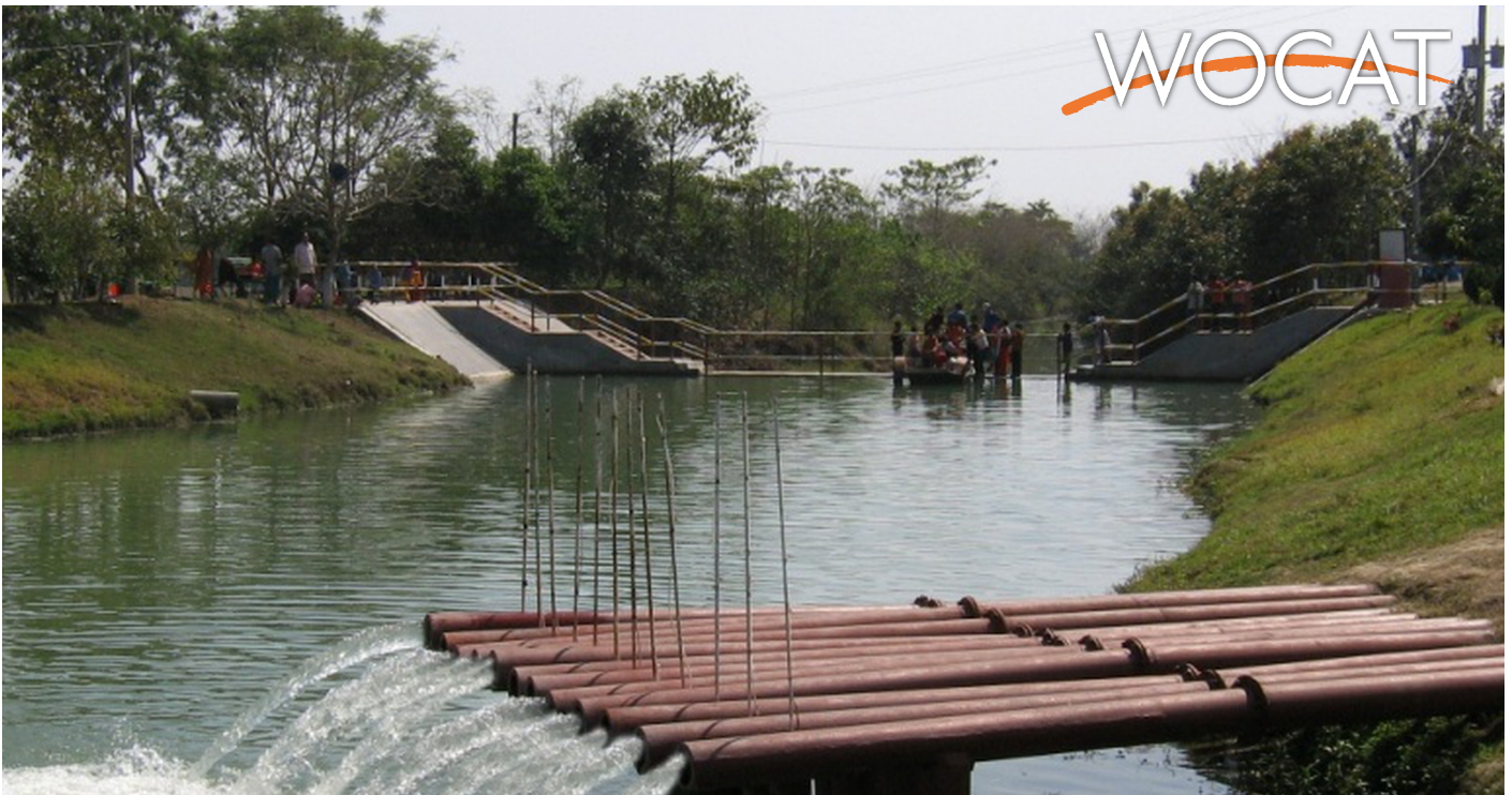
Water from the Padma river lifted to the Sharmongla canal for irrigation (Zillul Bari)
