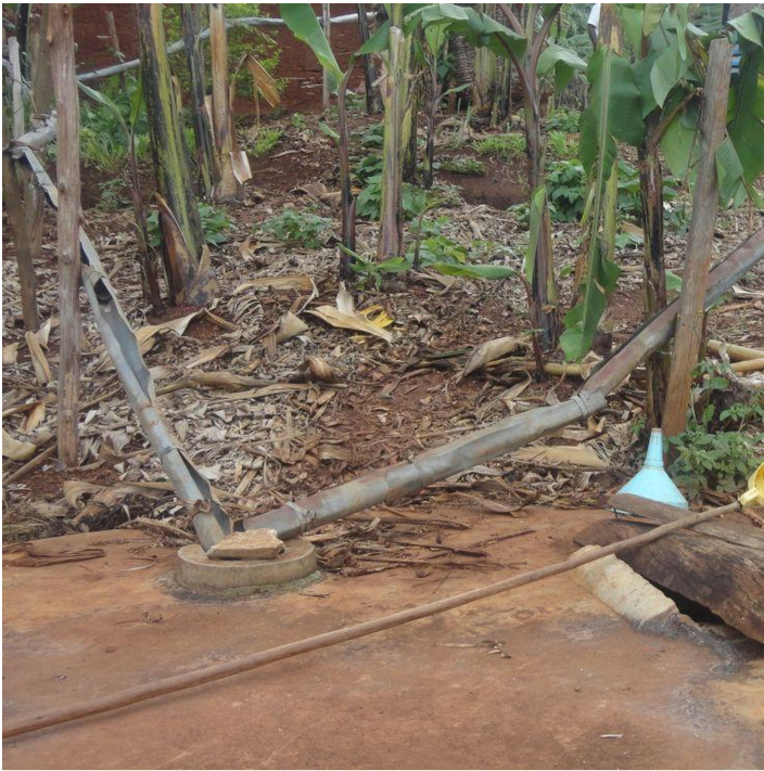
The storage tank capacity determines how long, during a dry spell, the farm household will stay water secure. A typical tank is 3m to 4m deep and 2.5m to 3.0m in diameter (Charles L Mlingu (Kagera TAMP, Kabale))
