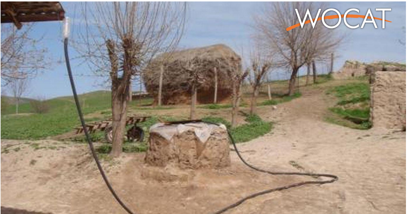
Low cost rainwater harvesting pond connected to the gutter with a pipe (Daler Domullojonov (14, Giprozem, app 27, Dushanbe, Tajikistan))
