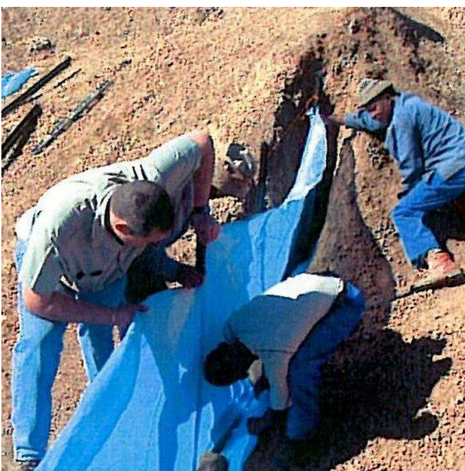
Soil erosion control
