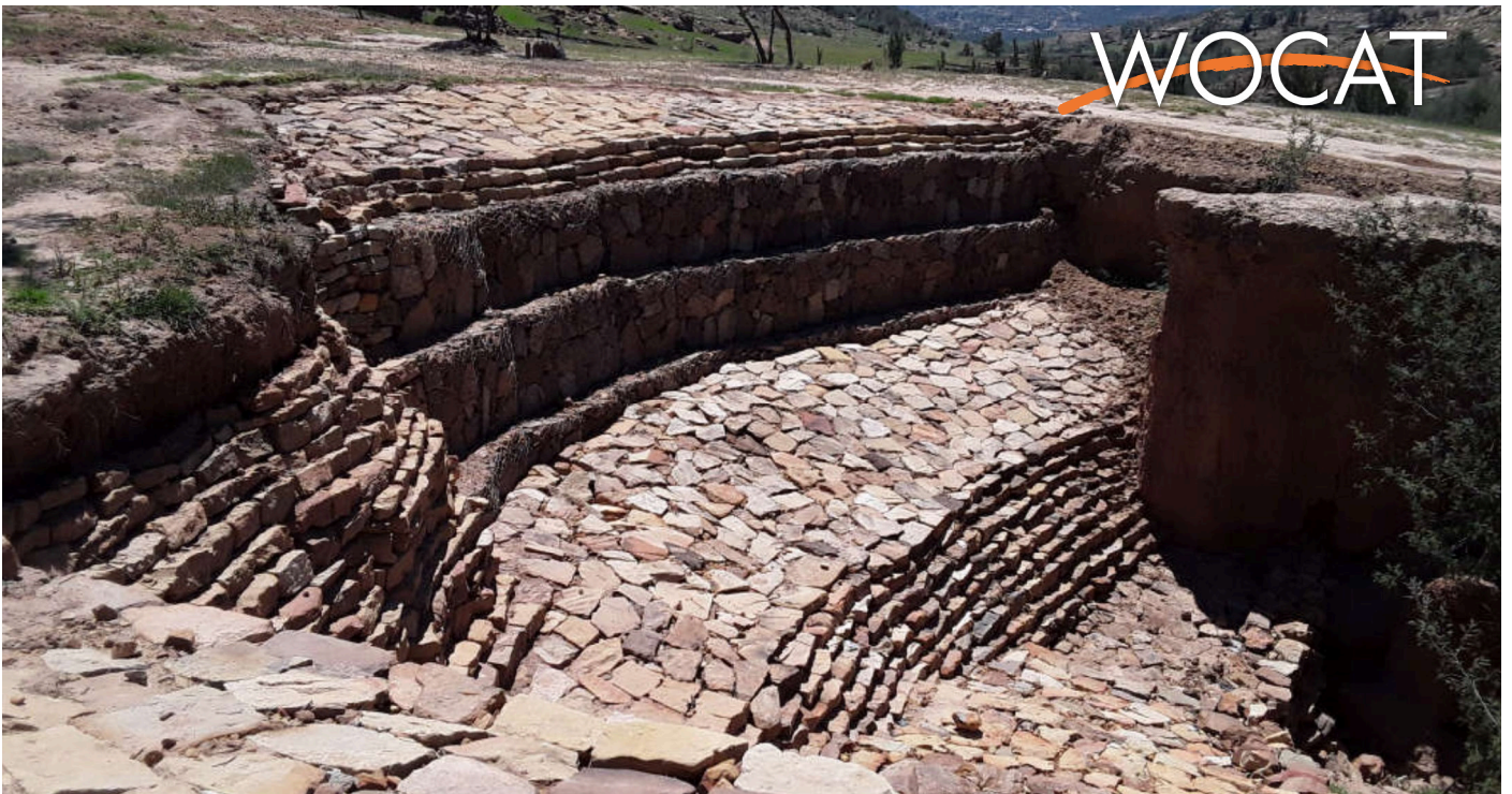
Gully head is constructed at the head of a gully using stones to discourage the gully from expanding further in length thereby stabilising the gully. (Koetlisi Koetlisi)
