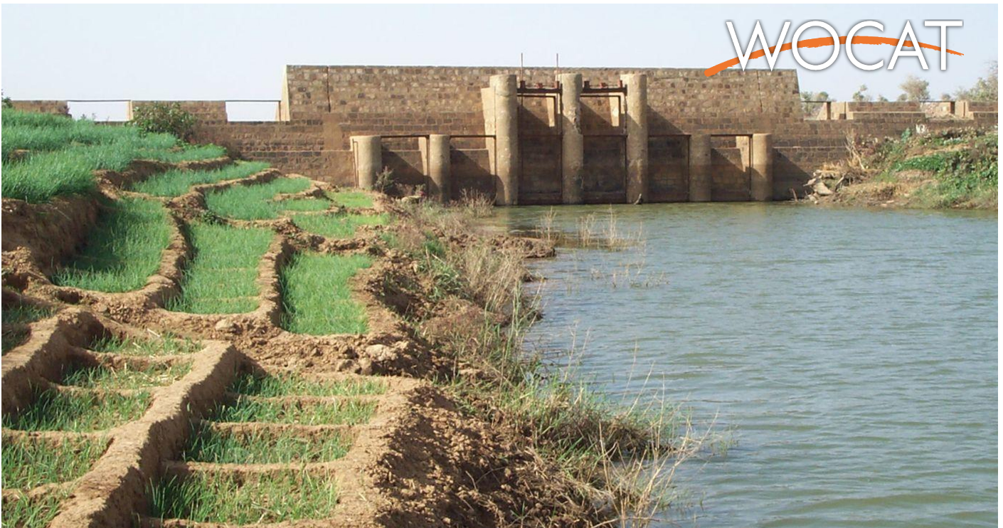
Masonry dam (PIPRO-DB)
