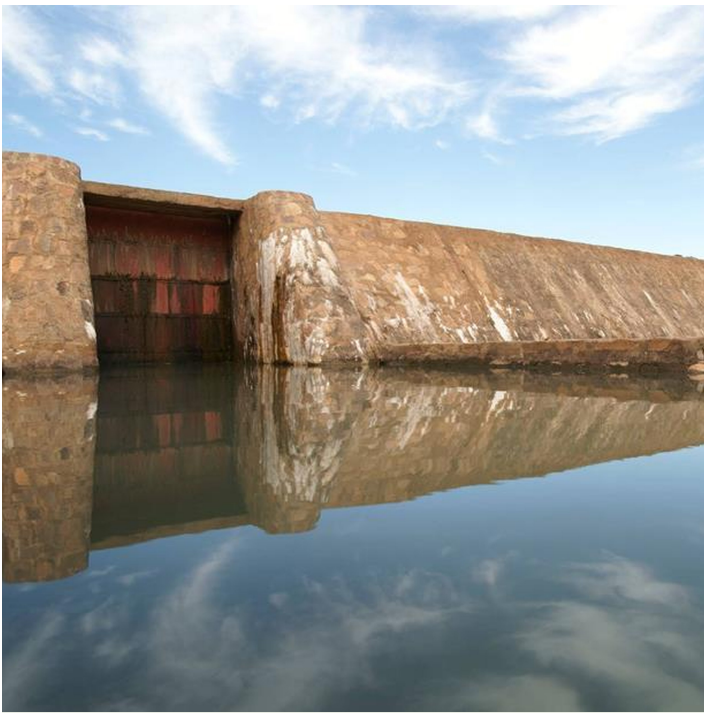
Masonry dam (PIPRO-DB)
