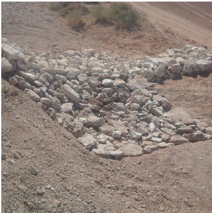
Gully plug construction (Mira Haddad)
