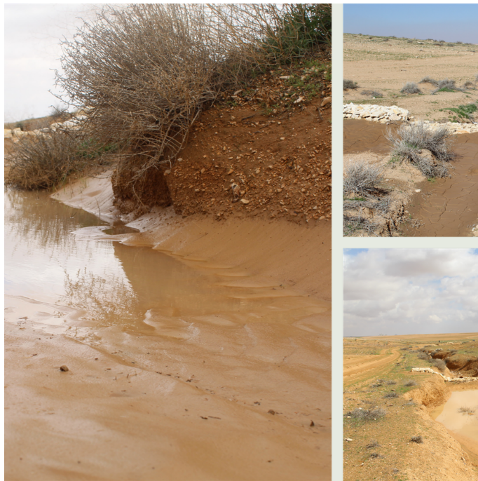
Gully plugs during the first rainy season 2017/2018. Photo looking downstream at the top of a gully plug with water ponded and sediment trapped upstream. (Mira Haddad)
