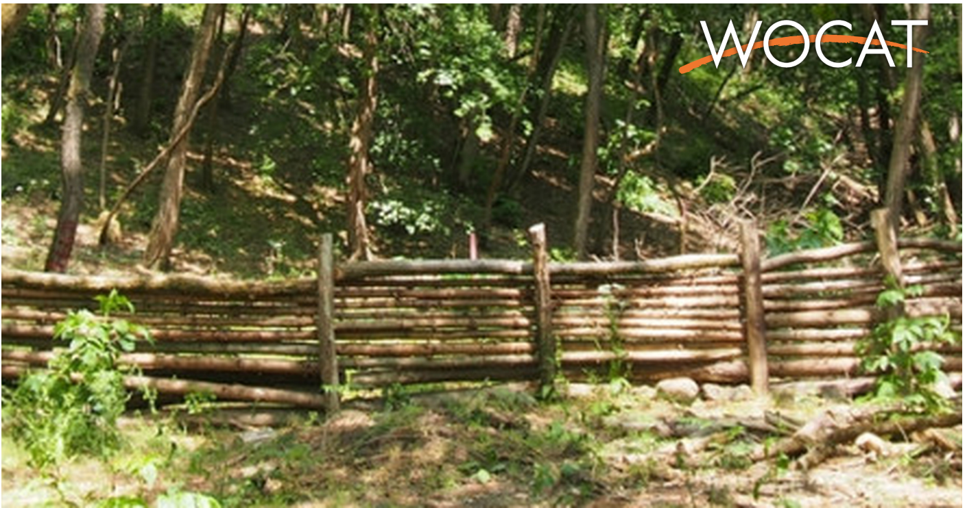
Water slowing leaky dam in the forest area of Püspökszilány (Klára Kerpely (source: https://wwfcee.org/news/five-hungarian-local-municipalities-lead-the-way-in-tackling-climate-change ))
